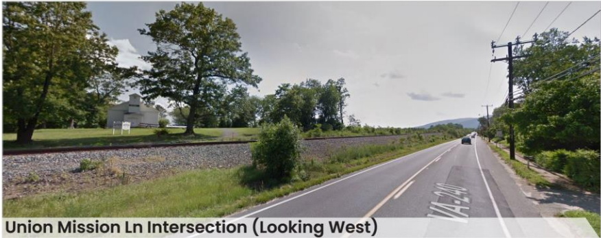
Union Mission Ln Intersection (Looking West) Just east of Union Run Ln., the Union Run Baptist Church (constructed ca. 1913 of rusticated concrete block) is visible beyond the railroad tracks and a view of the mountains opens up to the west.
