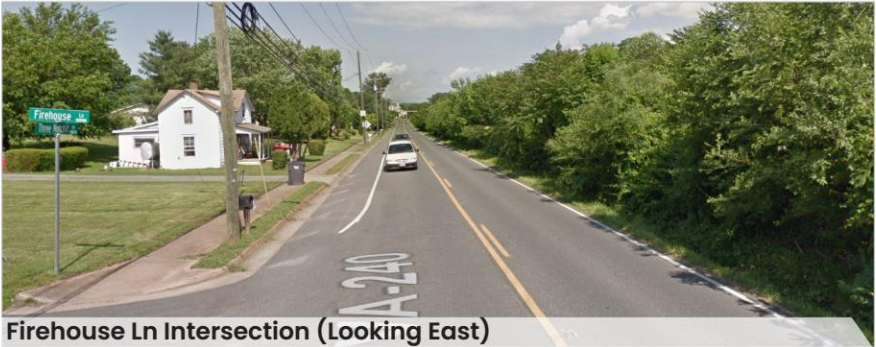
Firehouse Ln Intersection (Looking East) At Firehouse Ln. looking east, the railroad and roadside vegetation form a dense visual buffer on the south side. Small-scale residences from the first half of the twentieth century predominate on the north side.
